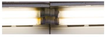
Existing lighting prior to relamping: Discolored, cracked coatings and brittle end caps on tube guards deems protective mechanisms ineffective for glass containment.
